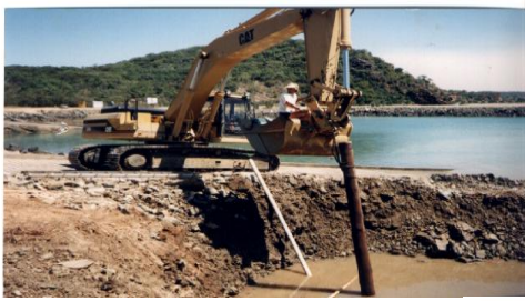
Driving piles, new hard stand & jetty
