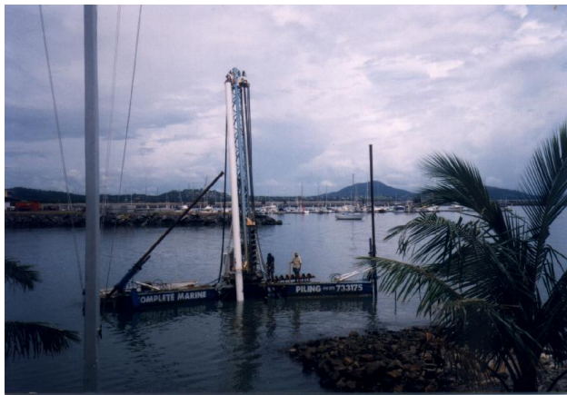
Driving the piles for pontoon,...
